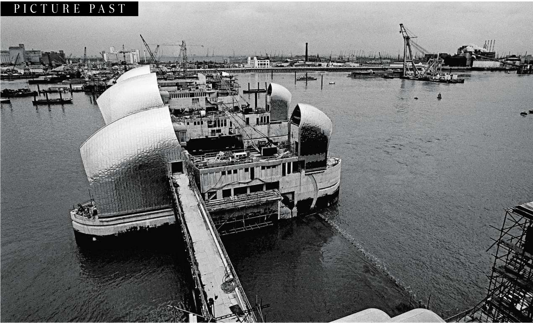
BEST DEFENCE: The Thames Barrier pictured under construction on the River Thames on July 7, 1980. Work began on the barrier in 1974 and it came into operation in 1982.
